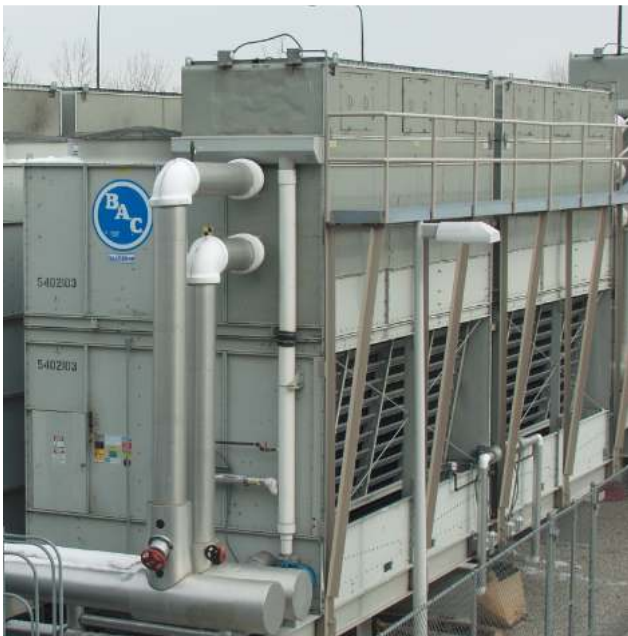
FIGURE 6: TYPICAL CLOSED CIRCUIT COOLING TOWER WITH PCD HOOD TO REDUCE HEAT LOSS IN COLD WEATHER [10]
