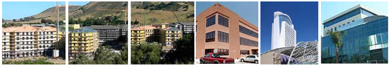
Photos of projects plan-checked or inspected by Willdan
