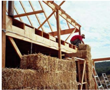
Straw Bale Construction
