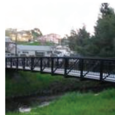
City of Pinole Prune Street Pedestrian Bridge Replacement
